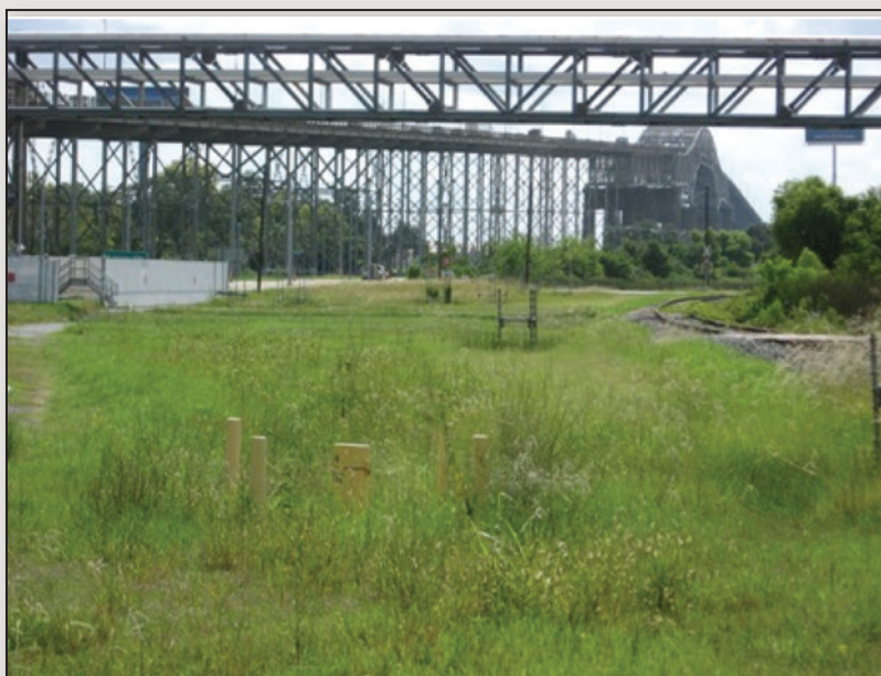
Area of planned remediation of soil and groundwater near proposed bridge and interchange construction.
